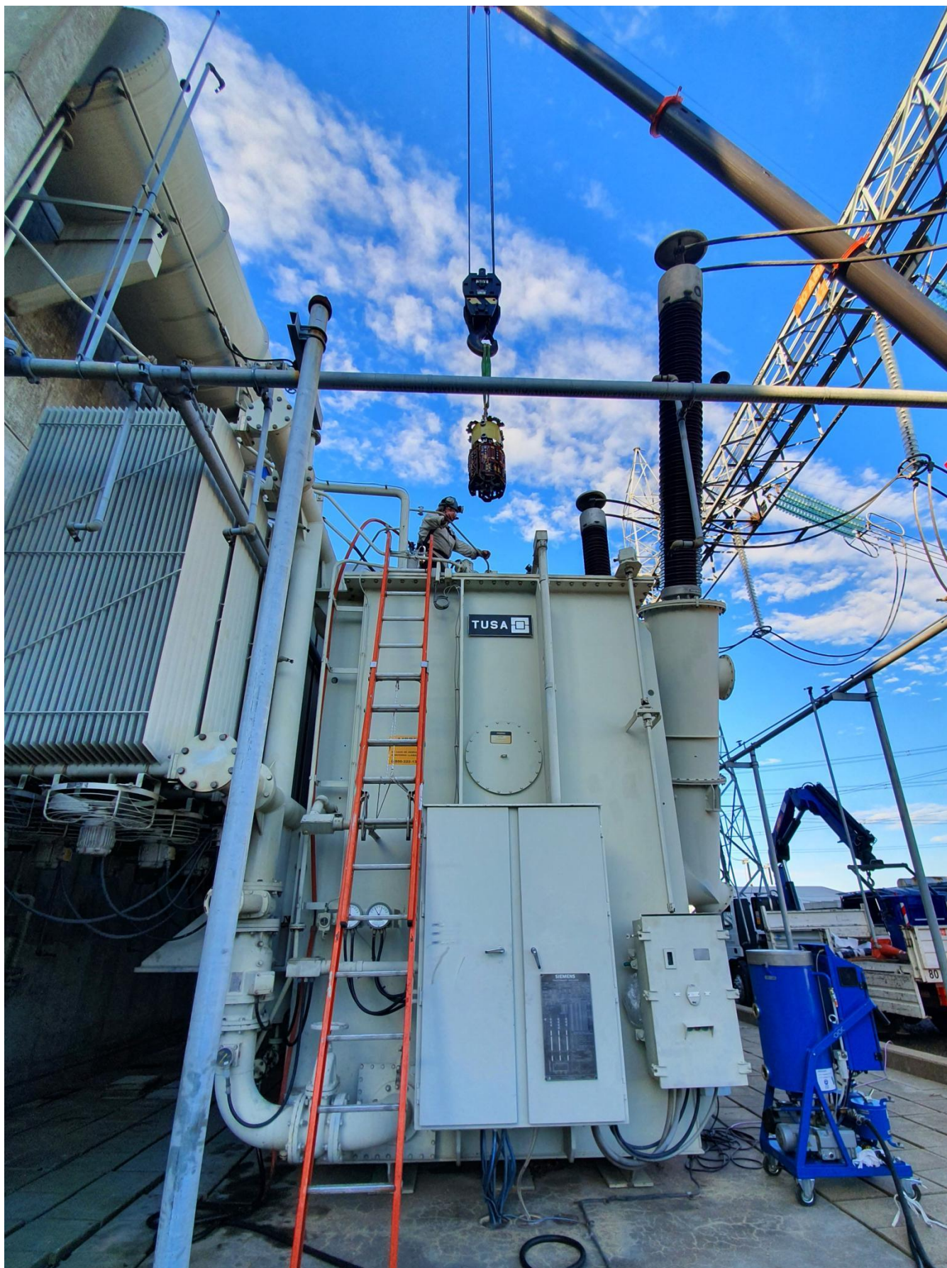
Big transformer and small 600 l/h transformer oil purification plant.
