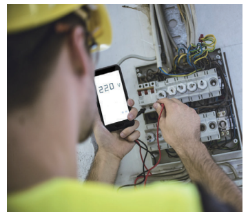
Electric Power Inspection
