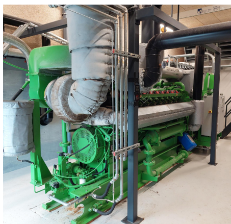
CHP engine unit at Haerup Biogas.
