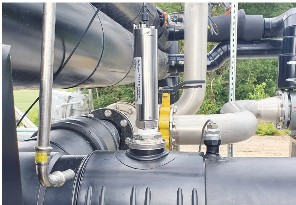
The SulfiLogger™ H 2 S sensor at Haerup Biogas. It measures in-pipe right after the biofilter.
