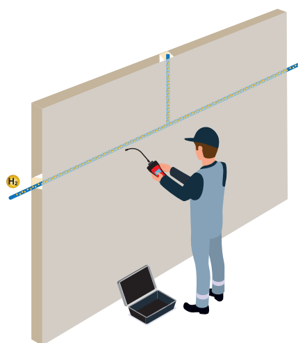
Tracer gas process on a water pipe
