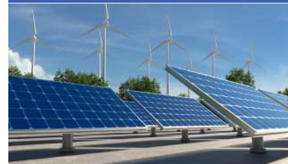
Renewable power converters
