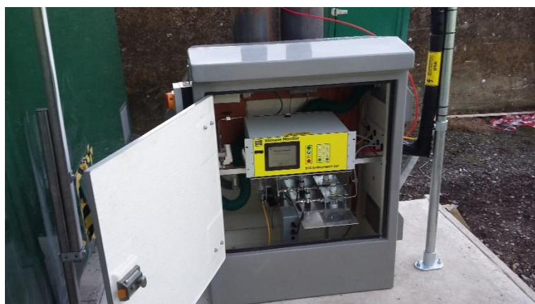
Siloxane Monitor package housed in GRP Kiosk
