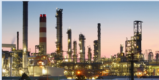
Down-hole power supplies (gas & oil)
